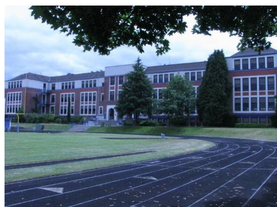
North (main) elevation of main building (118A) with track in foreground
