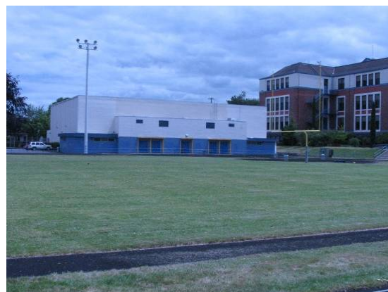
Looking southeast toward 1964 gymnasium.
