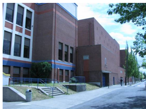
View of 1952 auditorium addition, looking south.
